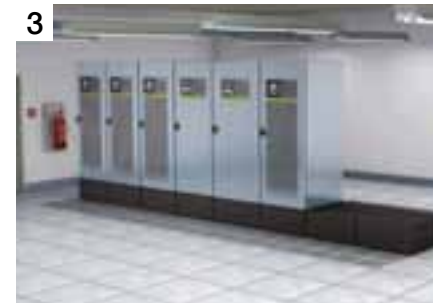
3 30 minutes later: 800 kW, online double conversion mode
